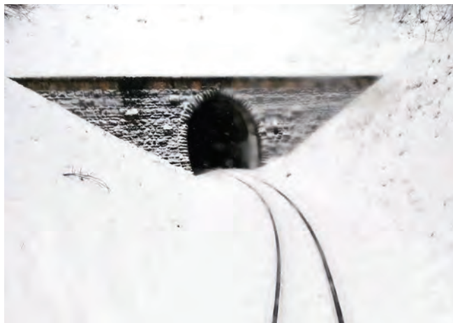
In contrast, a snowy day during the recce trip showing the portal of the curved Children's Railway tunnel.
